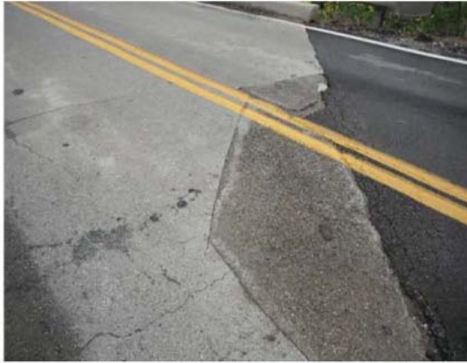
Deck has multiple patches/cracks/delaminated
