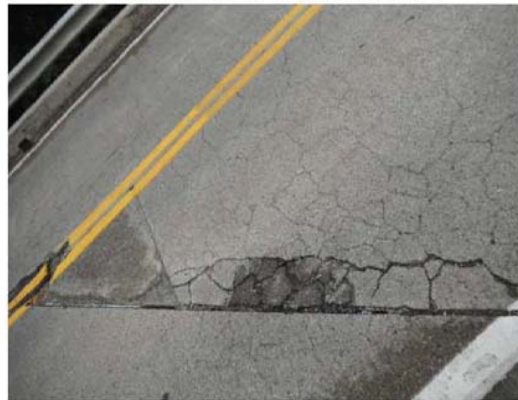
Cracked and delaminated areas breaking up along joint
