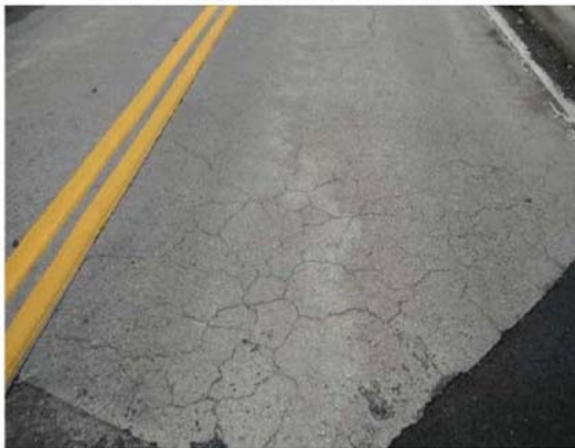
Deck cracks w/delamination
