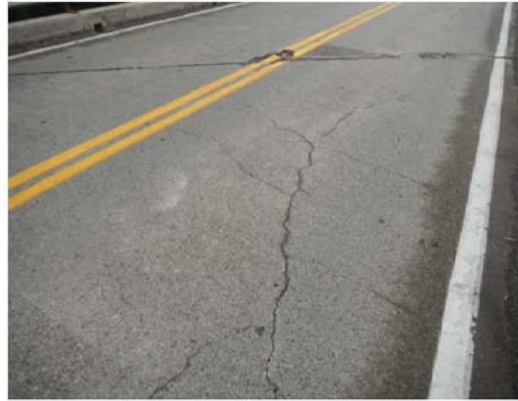
Deck has lots of cracks w/delamination
