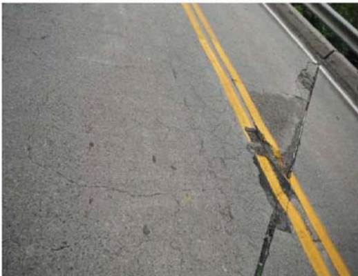
Deck spalling and breaking up along joint
