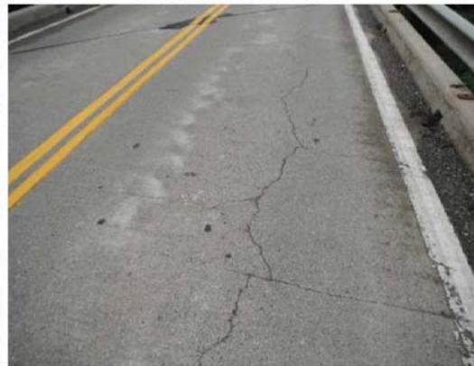
Deck cracks w/delamination
