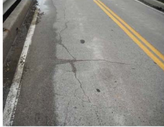
Deck cracks w/delamination
