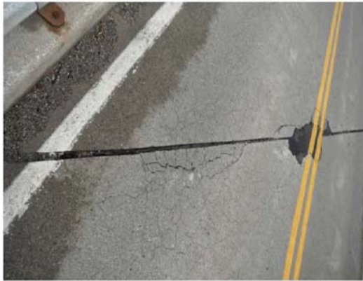
Cracked and delaminated areas breeking up at joint
